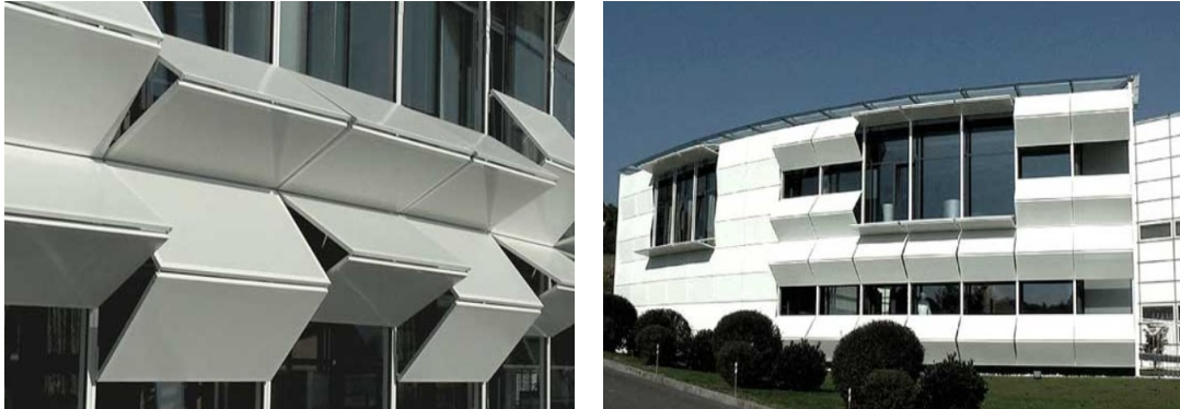
Figure 3: Kiefer Technic Showroom in Austria ( http://www.facade-interior.com ).
